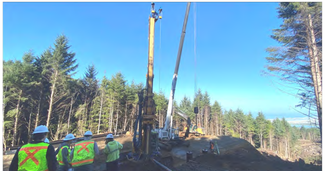
Soldier pile wall progress
