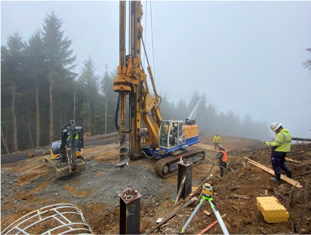
Drilling the shafts for the piles
