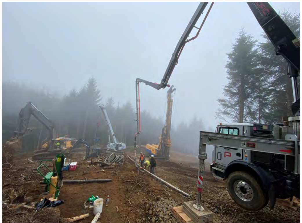
Pouring concrete in the drilled shafts
