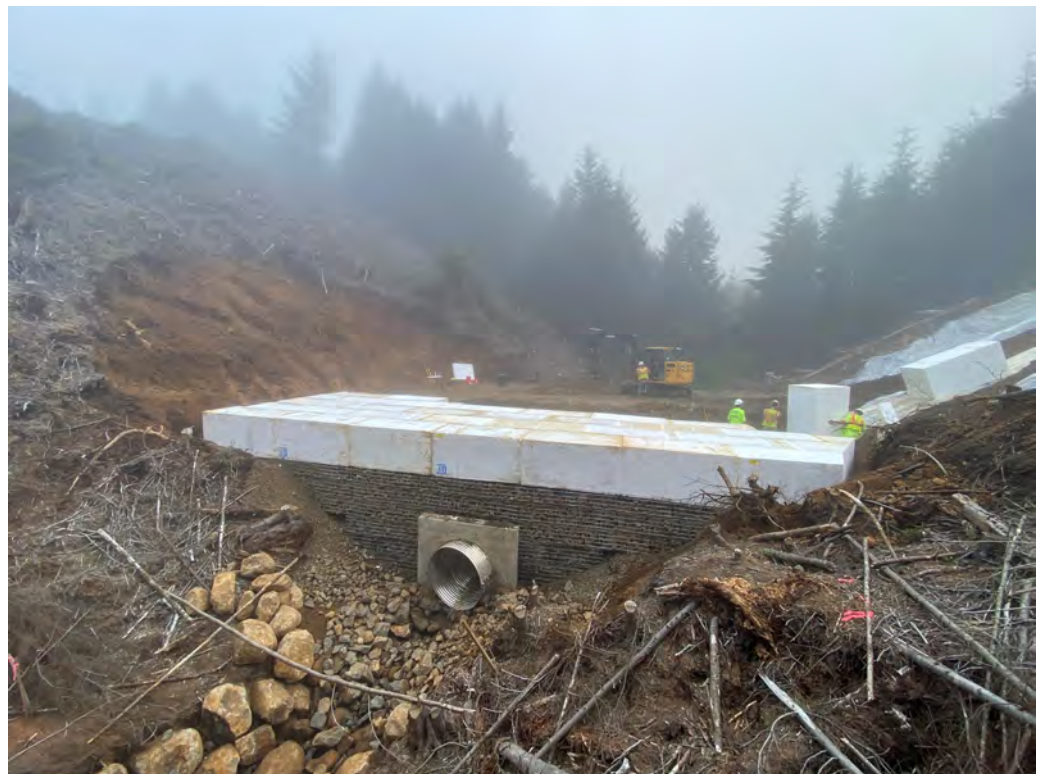
Installing geofoam blocks for the first row
