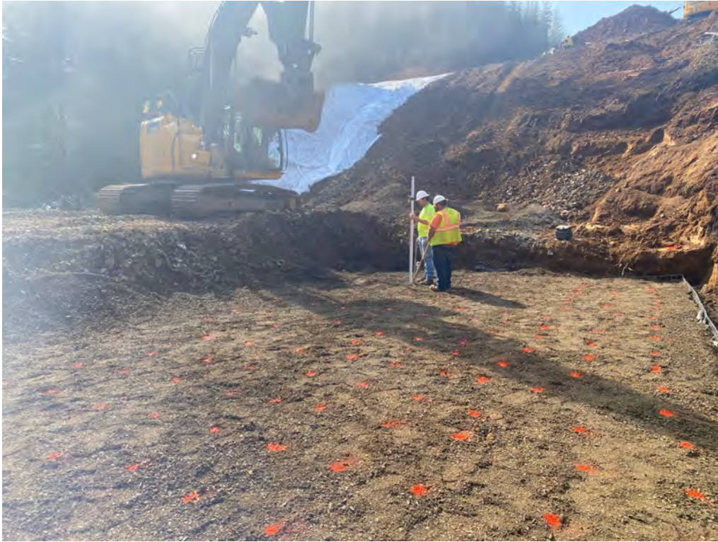
Preparing MSE wall surface for the Geofoam wall
