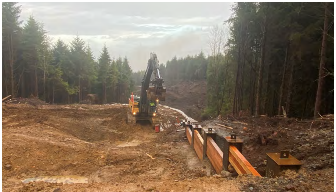
Timber lagging partially installed on the piles
