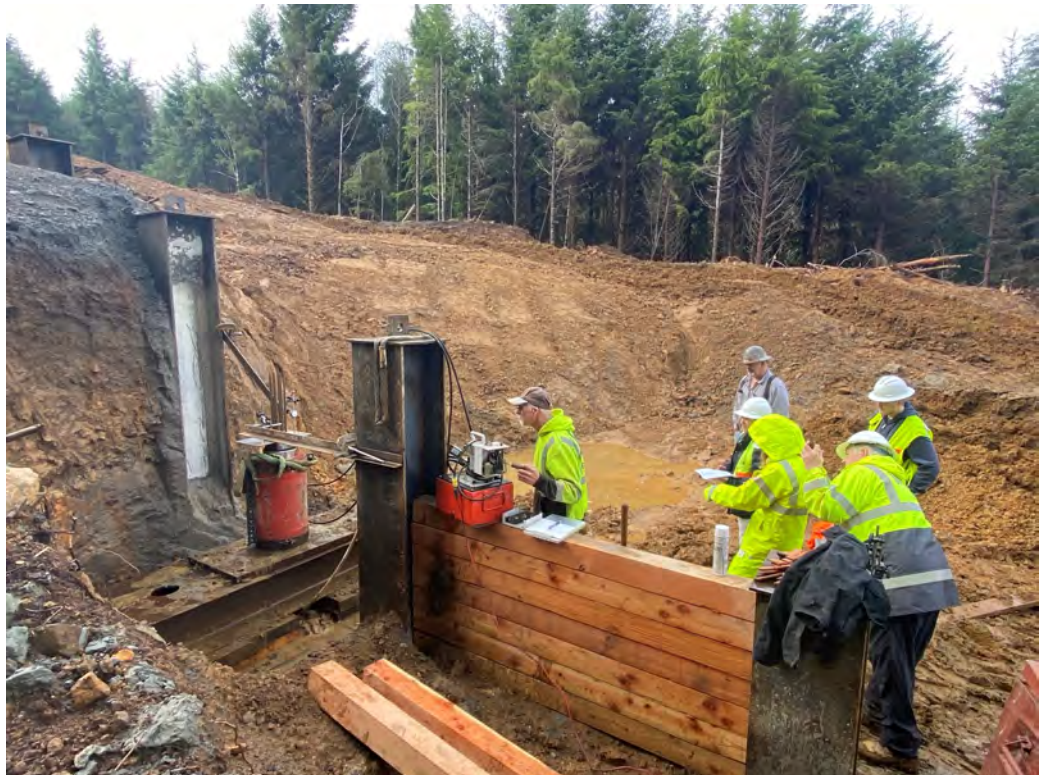
Ground anchor testing
