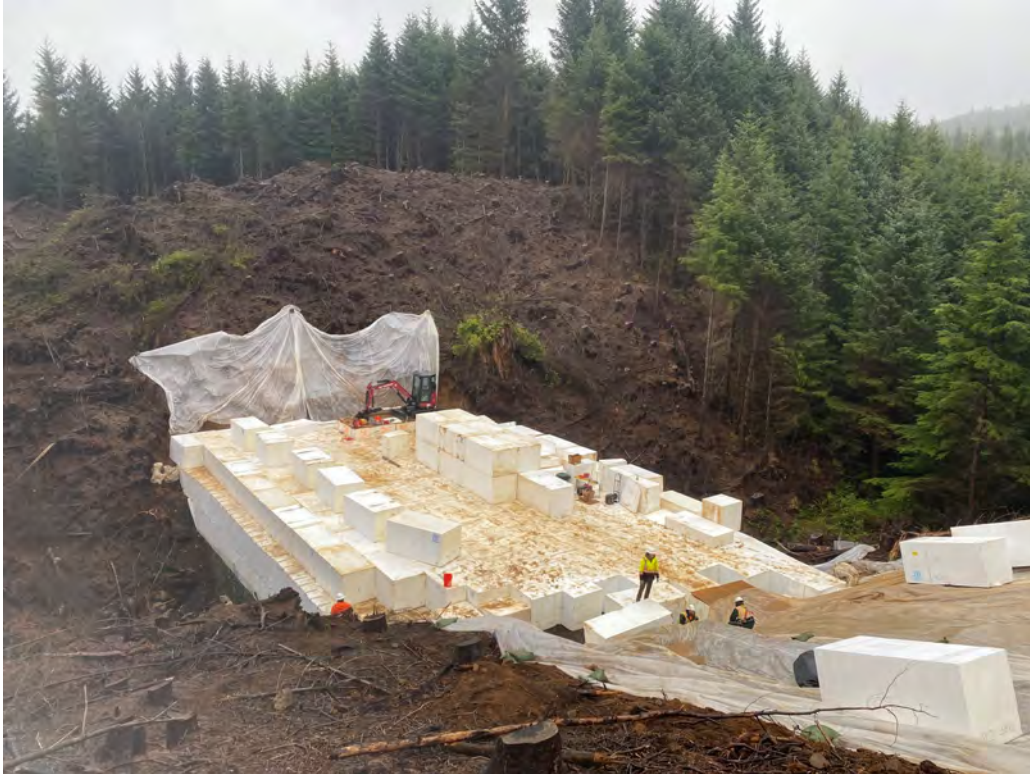
Geofoam wall progress
