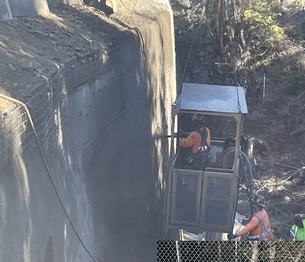
View of last day of shotcrete application.
