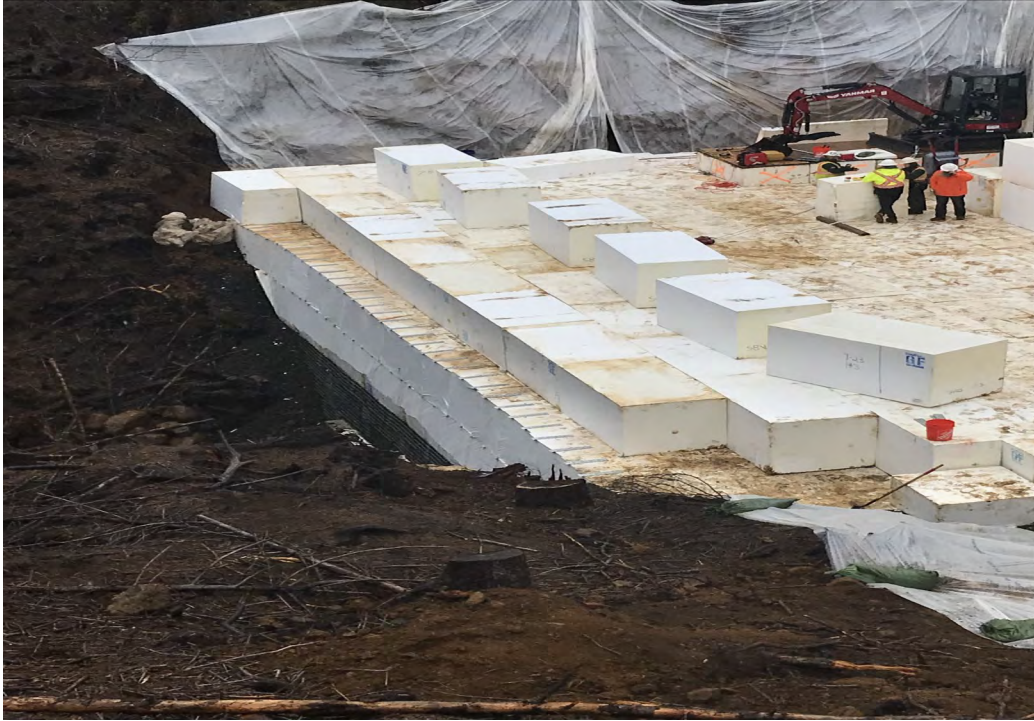
Geofoam wall pro- gress
