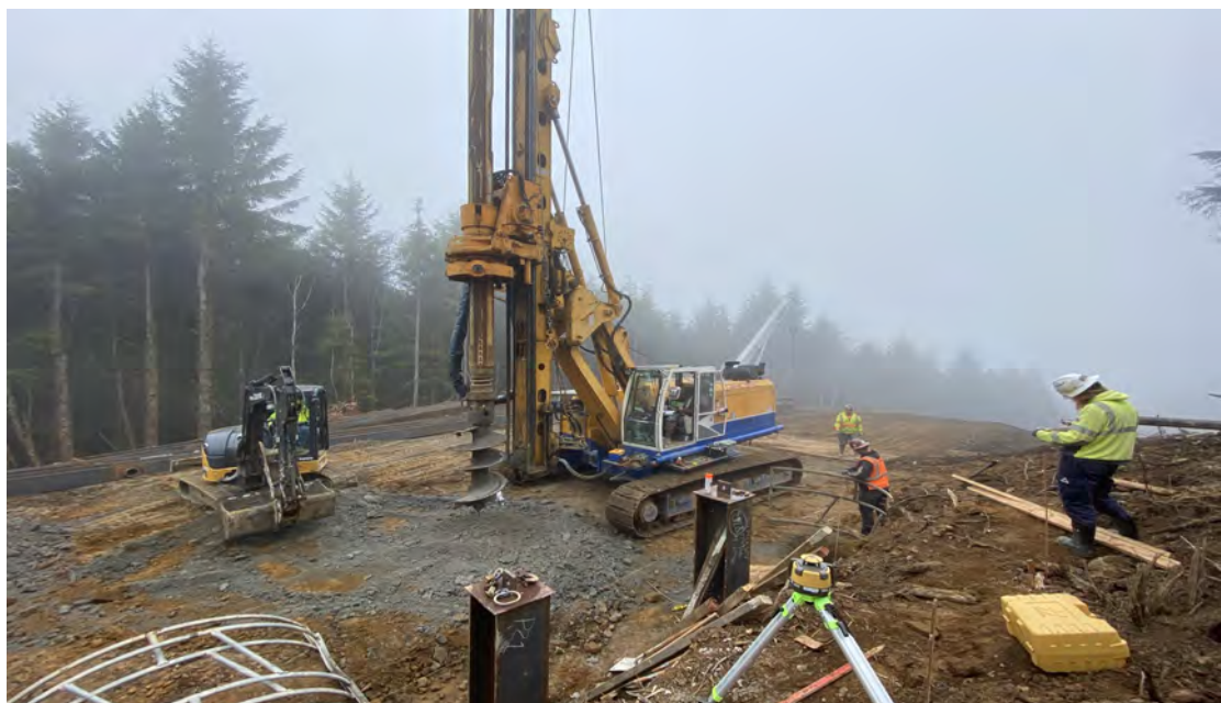
Drilling pile shafts in the fog
