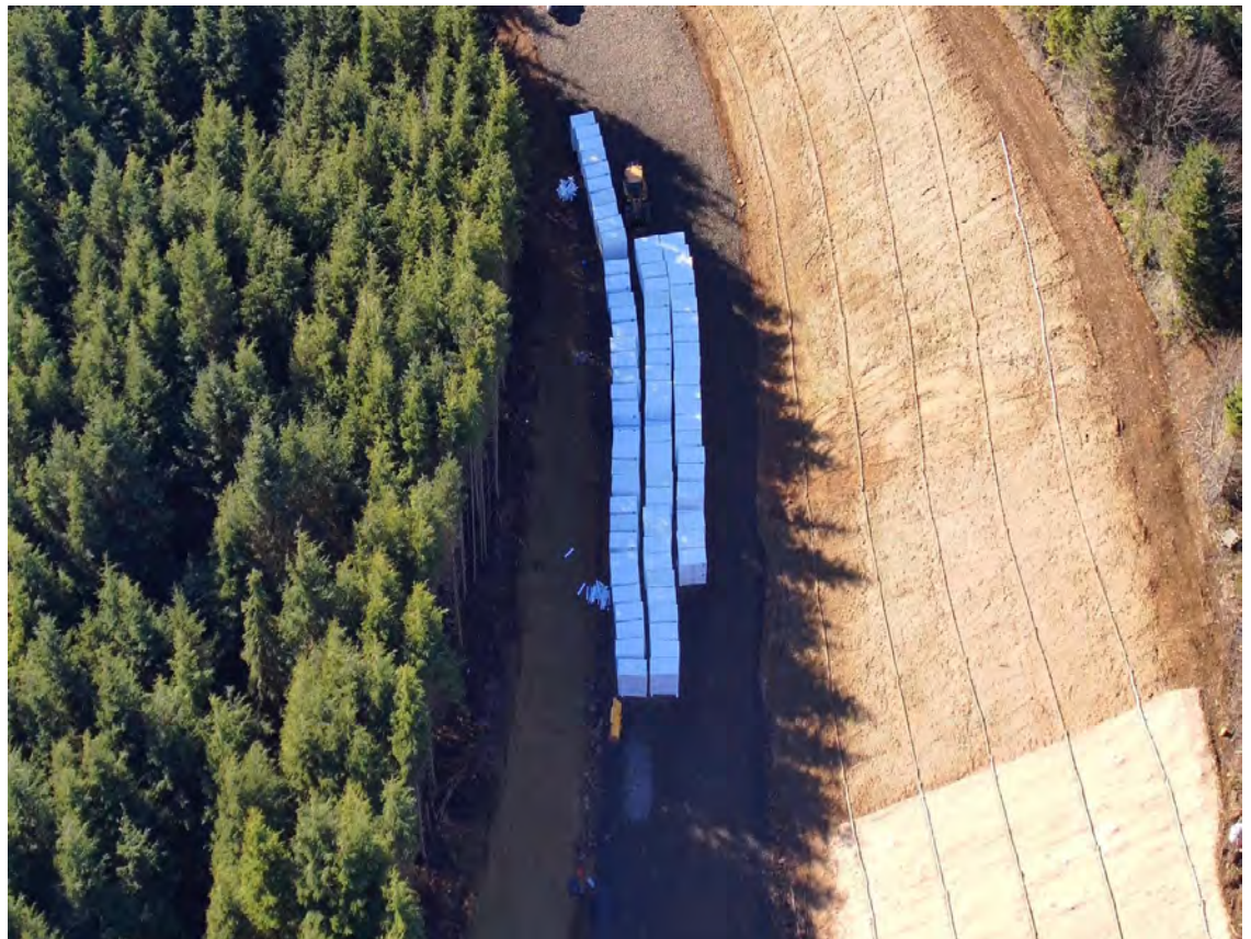
Geofoam blocks staged for installation.
