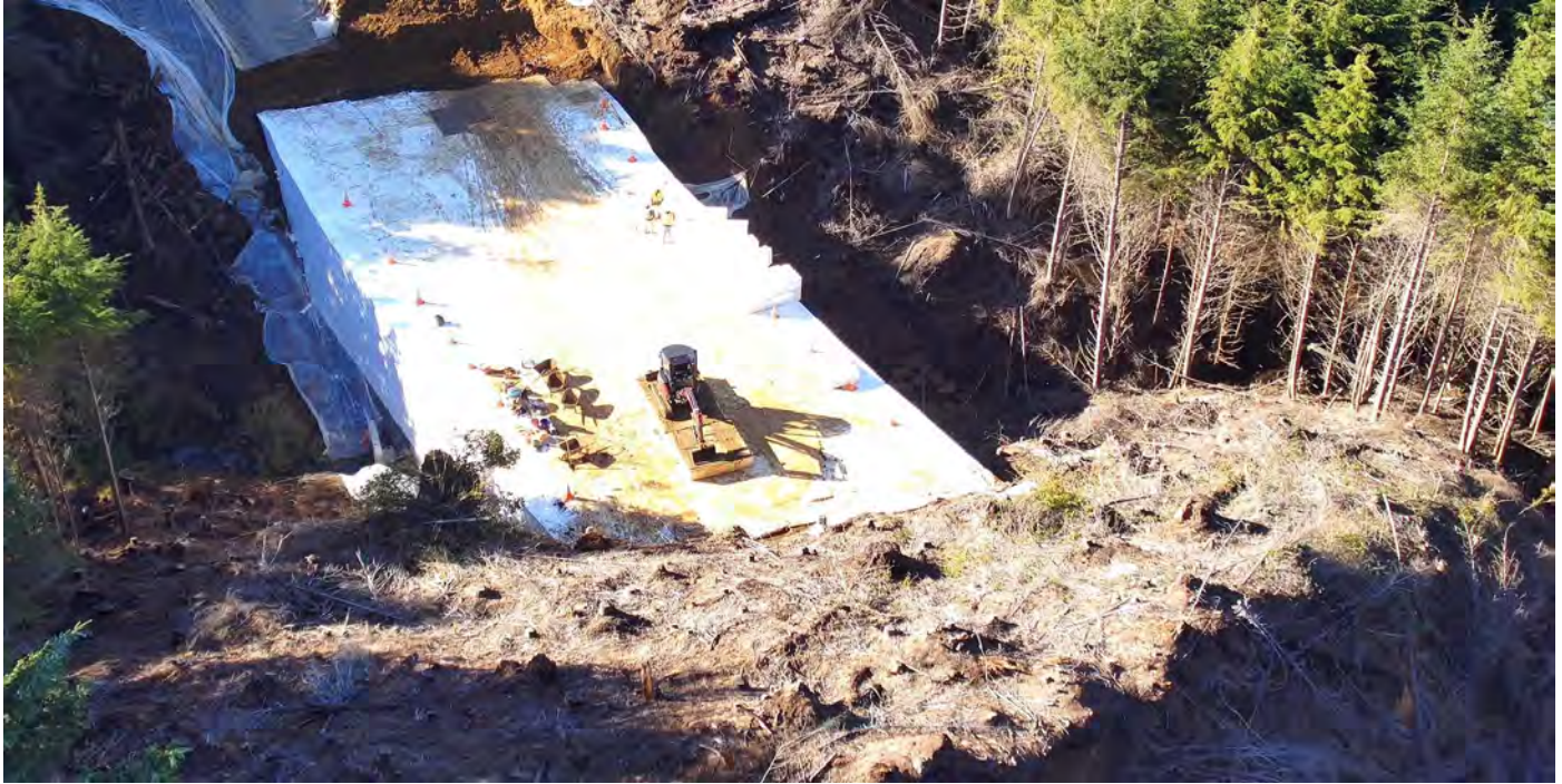
Geofoam wall progress
