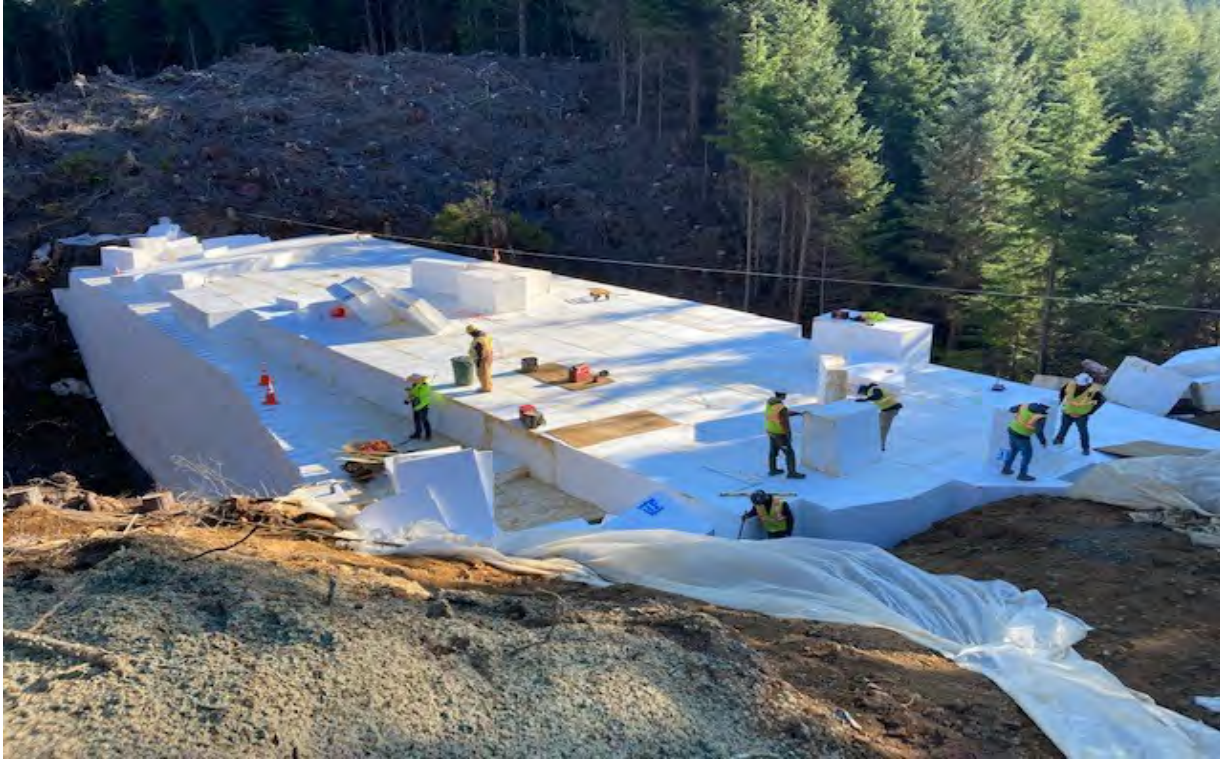
Geofoam wall progress
